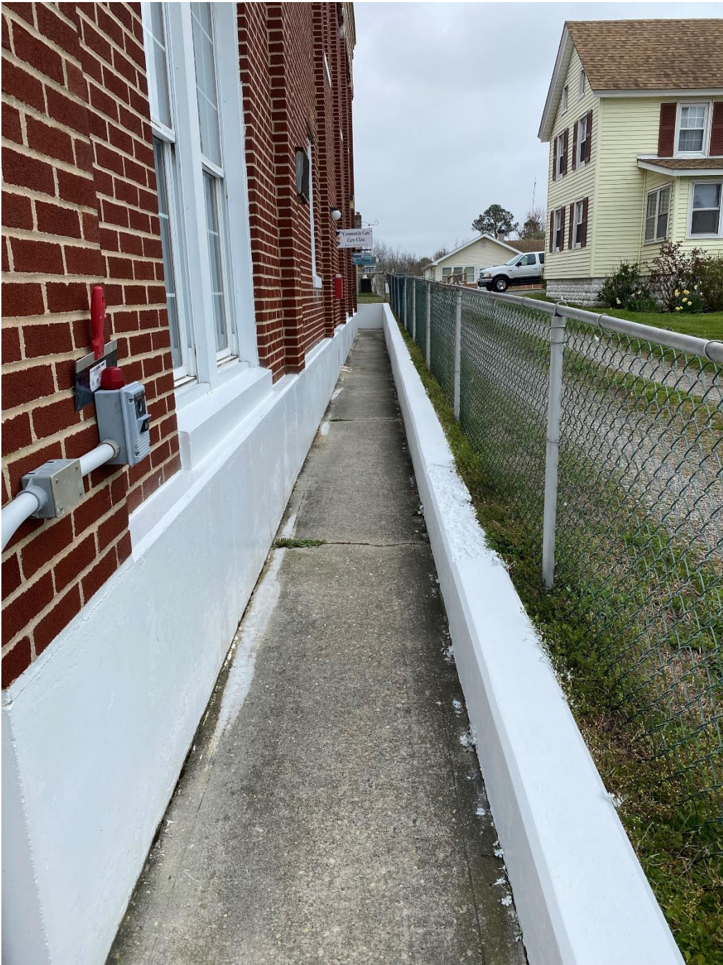
Old fire house maintenance including cleaning, painting, lights and screens.
